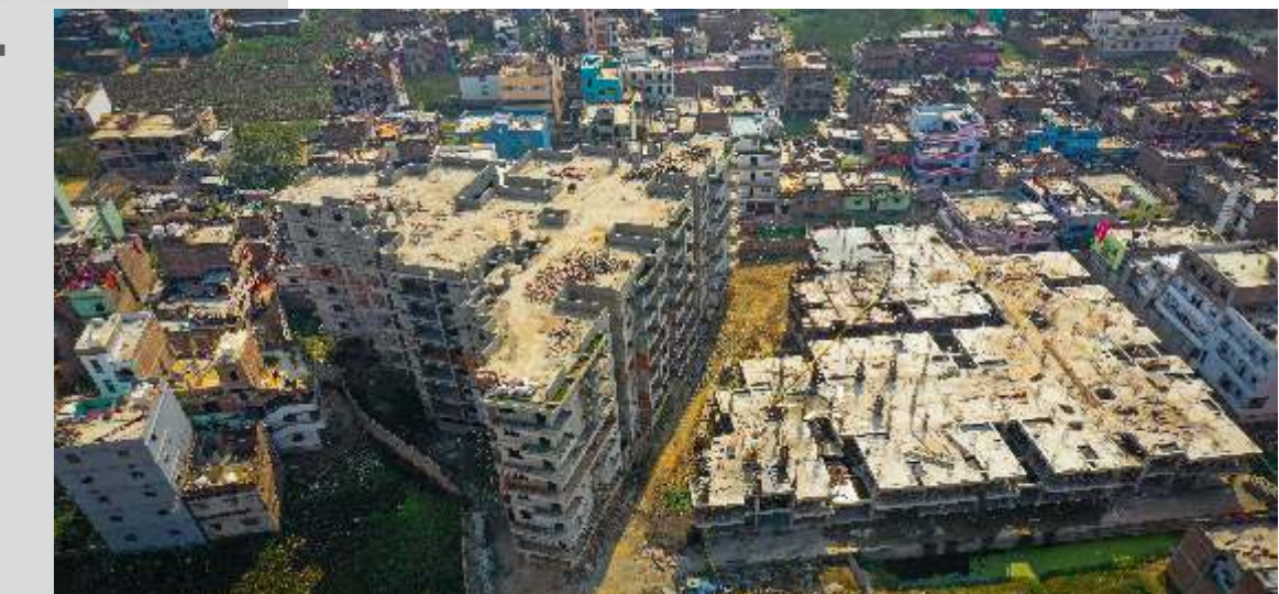
On going project The 7 planet Bhupatipur Mithapur bus stand
